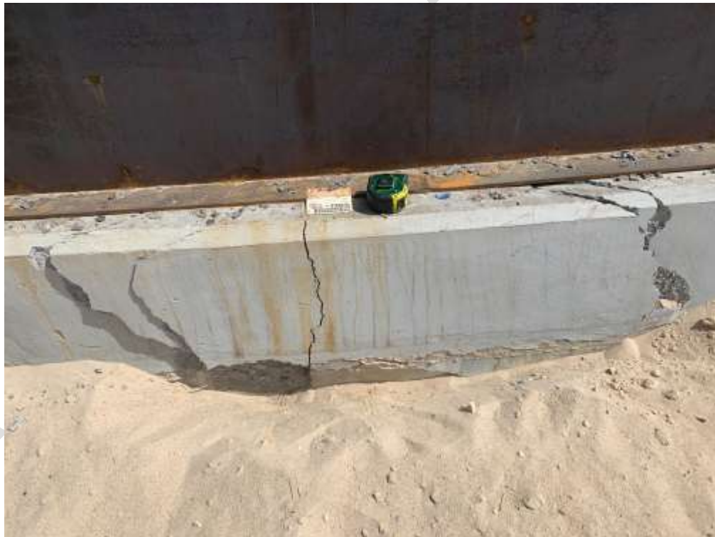
Figure 2- This photograph shows the result of not having the ringwall notched. The groove worn during construction caused outside edge of the back-up bar to "catch" and when the bottom/tank expanded, it caused a lateral loading on the top of the ringwall, thus spalling a large area.
