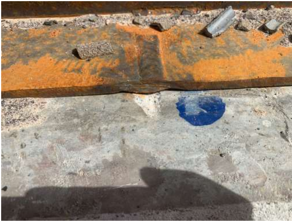
Figure 1 - Photograph shows a back up bar resting on a foundation without notches. This shows the groove that developed during construction due to thermal expansion and contraction.
